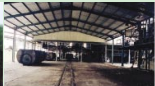
New extension transfer carriage station.
