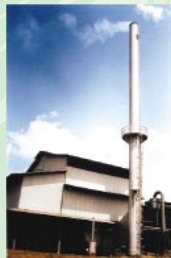
MHC-Kemayan mill new extension boiler station.
